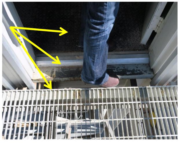
Transition between walking surfaces with a floor hole in between – trip hazards coming and going!
